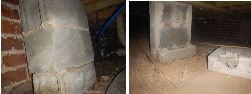
Pier (left) immediately inside access opening has broken mortar joint with upper section tilted off vertical. Pier under living room (right) is broken in half.
