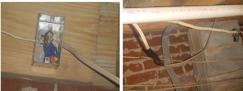
All line splices, wiring connections and abandoned wires should be enclosed in covered junction boxes. Also note metal seismic/wind lift control strap (right) that has not been attached to new wood of sill above.
