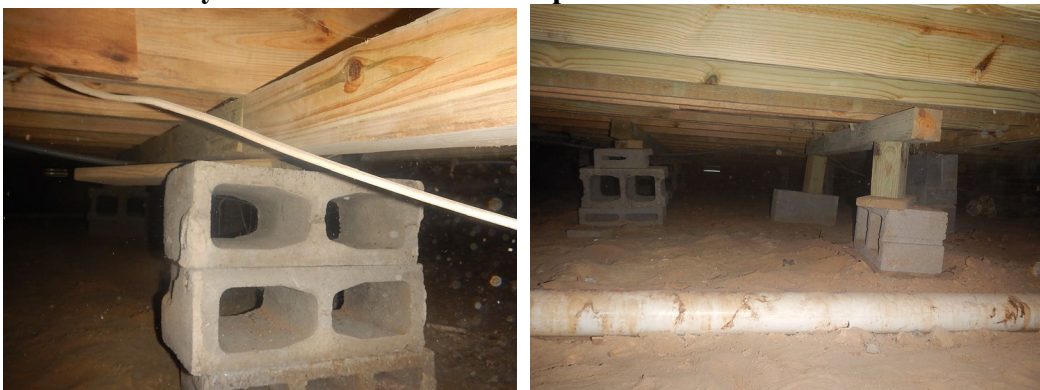
Improperly oriented (horizontal rather than correct vertical) orientation of cells makes blocks subject to failure. Short wood “Stiff Knees” are not stable supports (right). Also note scabbed floor joist repair (left) that can fail if not properly supported.
