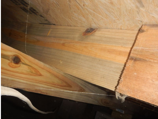
Example of scabbed repair with 4x4 support. Slight sagging has already occurred
