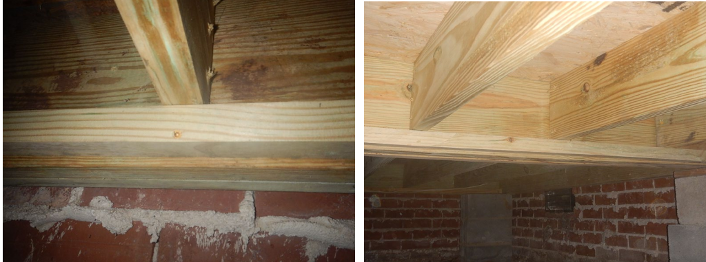
Ledger (left) with on screw under joist and toe-nailing visible. Random (right) spacing of tan color nails (hard to see screw heads in wood)
