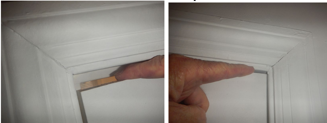
Latch side of door (left) has large gap at top when closed and hinge side (right) has normal gap
