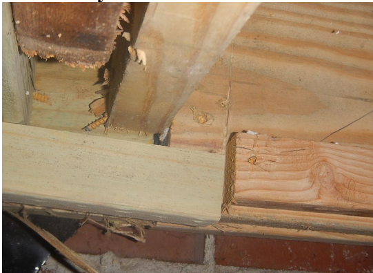
Example of sagging/misaligned butt jointed sills. Also note tan color decking screw used to toenail floor joist to sill
