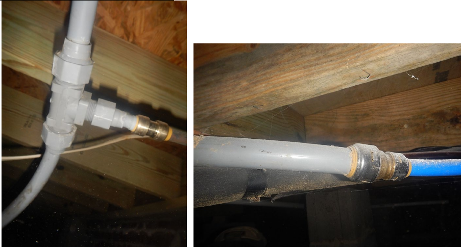
Examples of polybutylene gray pipe and connection to blue PEX cold water line
